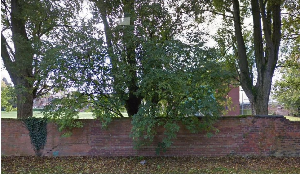
Boundary wall and trees looking south towards the northern gable end of the Mayfield building
